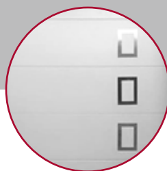
2. Geometrie in lamiera di acciaio inox satinato e incollate sui pannelli mediante speciali adesivi. Geometric shapes made of brushed stainless-steel and glued to panels using special adhesive material.
